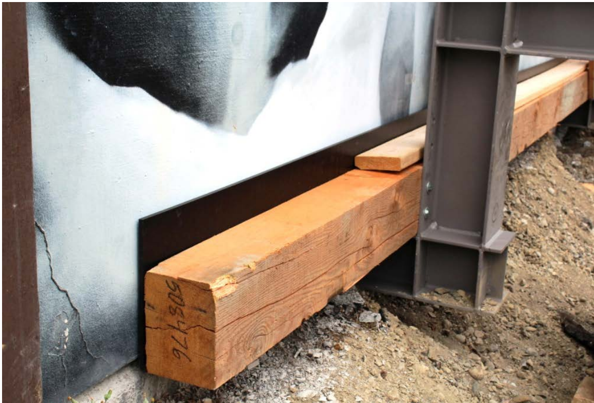
The A-frame in place from the front of the mural
