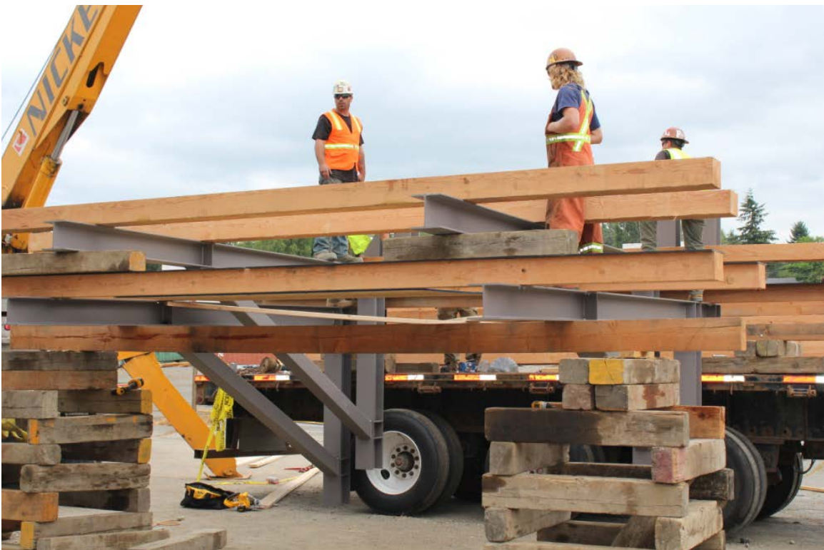
A total of 17 A-frames were constructed to move all 8 murals
