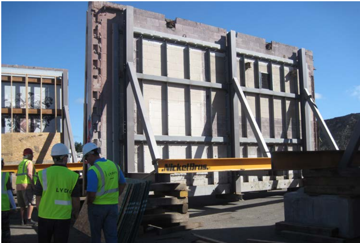
Steel reinforced backing was built into the CMU walls for added support
