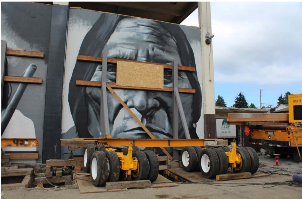
Hydraulic dollies ready to be attached to the A-frame for removal
