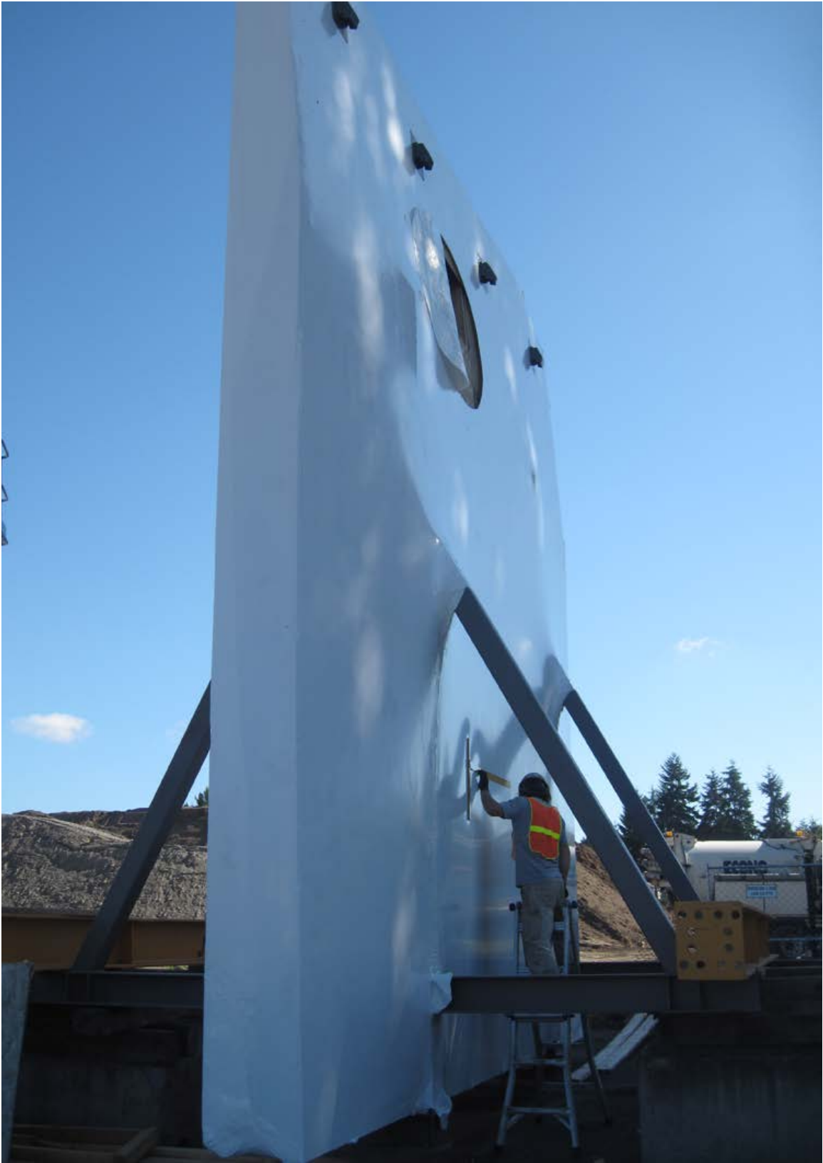
Industrial shrink wrap was applied to protect all murals after their removal
