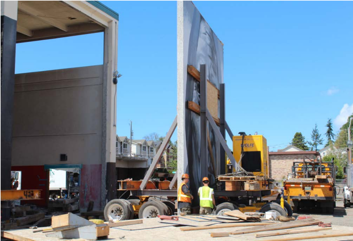
Hydraulic dollies were attached to both sides of the A-frames for all removals
