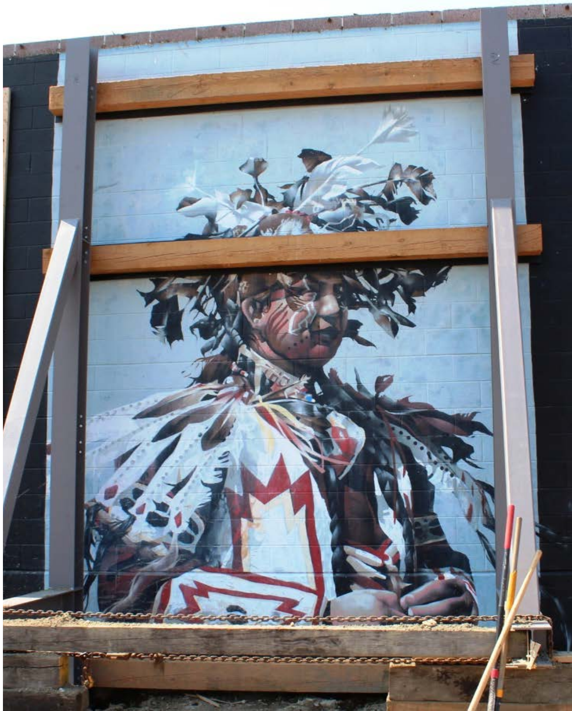
Chilliwack mural supported by A-frames
