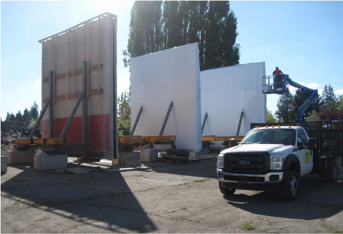
Walls being shrink wrapped for added protection
