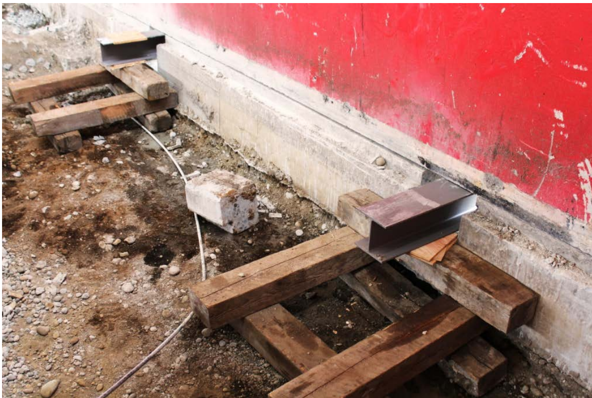
The A-frame in place from the backside of the mural
