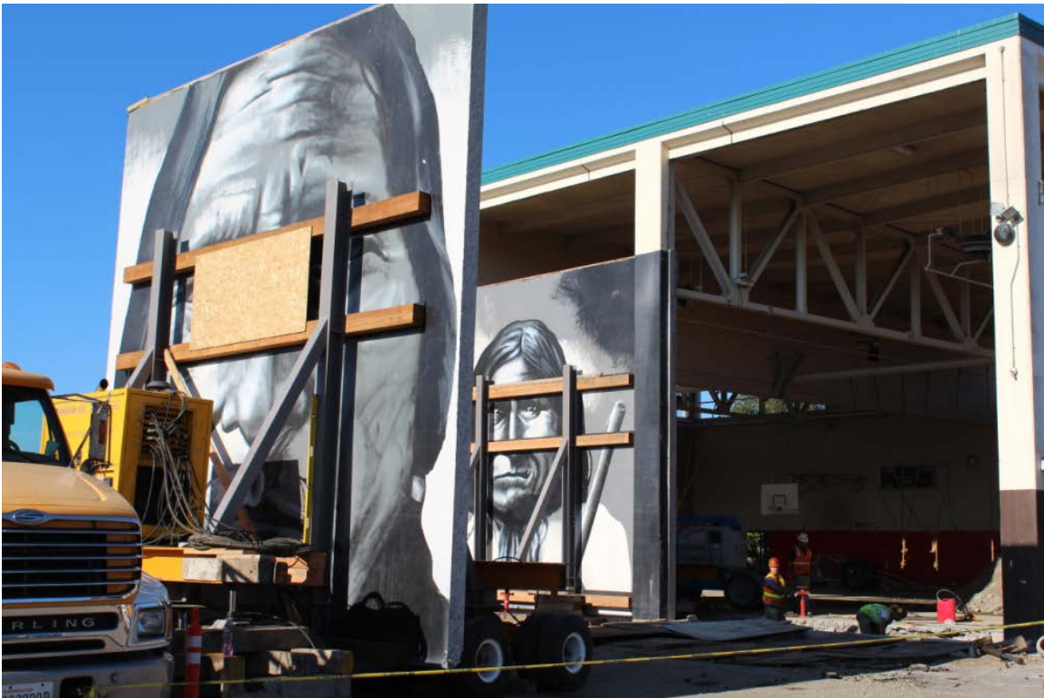
The hydraulic dollies were remote operated and controlled with a joystick
