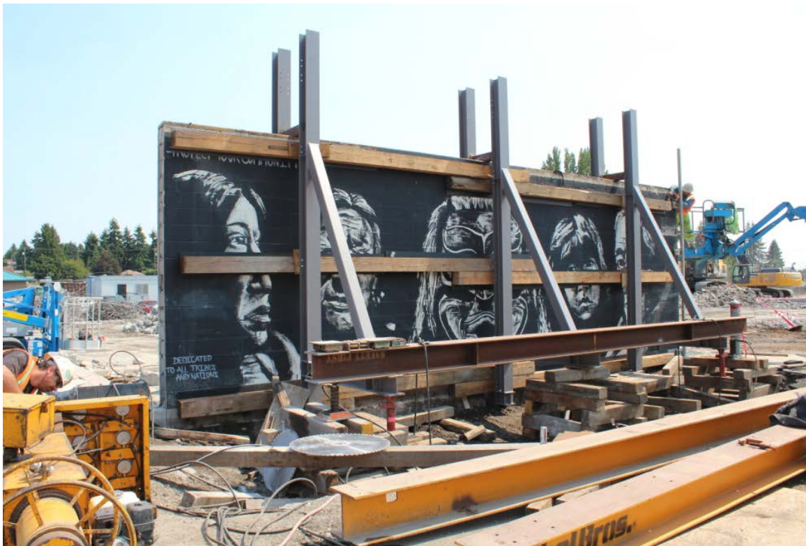
Longhouse mural supported by A-frames and ready for hydraulic dollies
