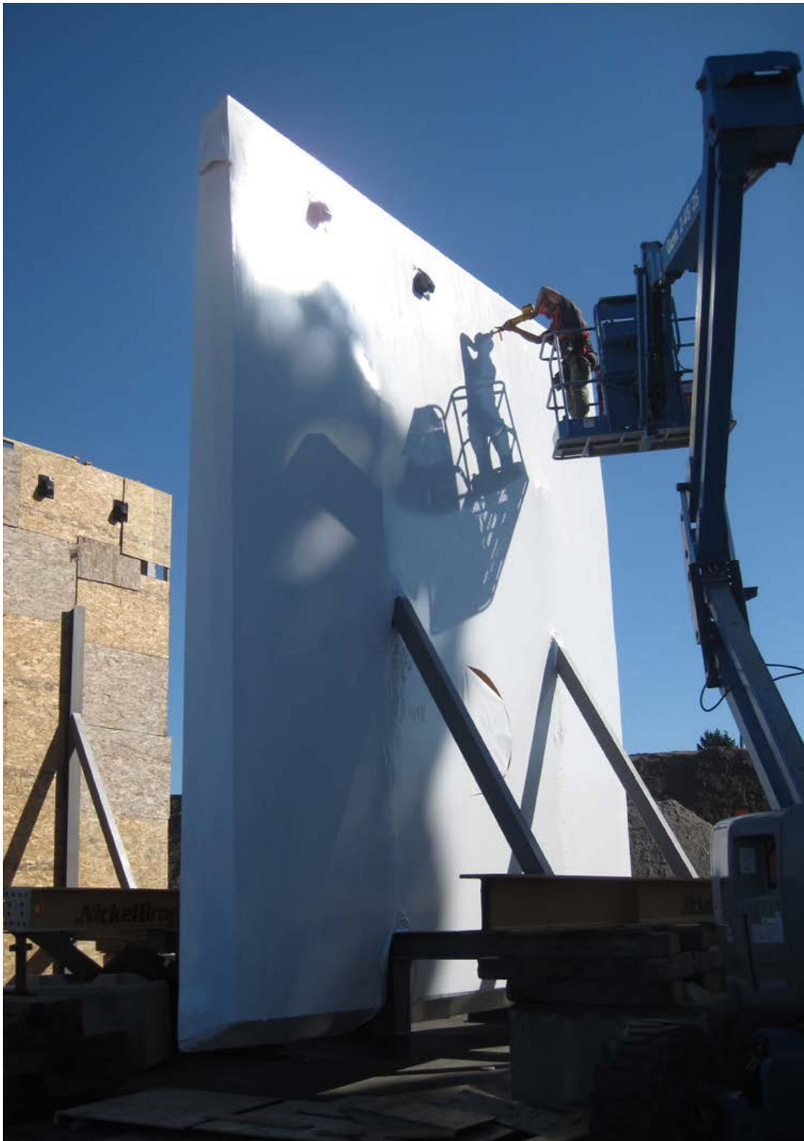
Ventilation and viewing windows were constructed into the plywood and industrial shrink wrap
