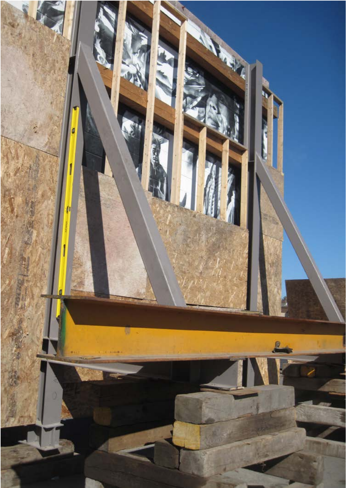
After the shrink wrapping, a plywood wall was then built on the face of the murals for added protection
