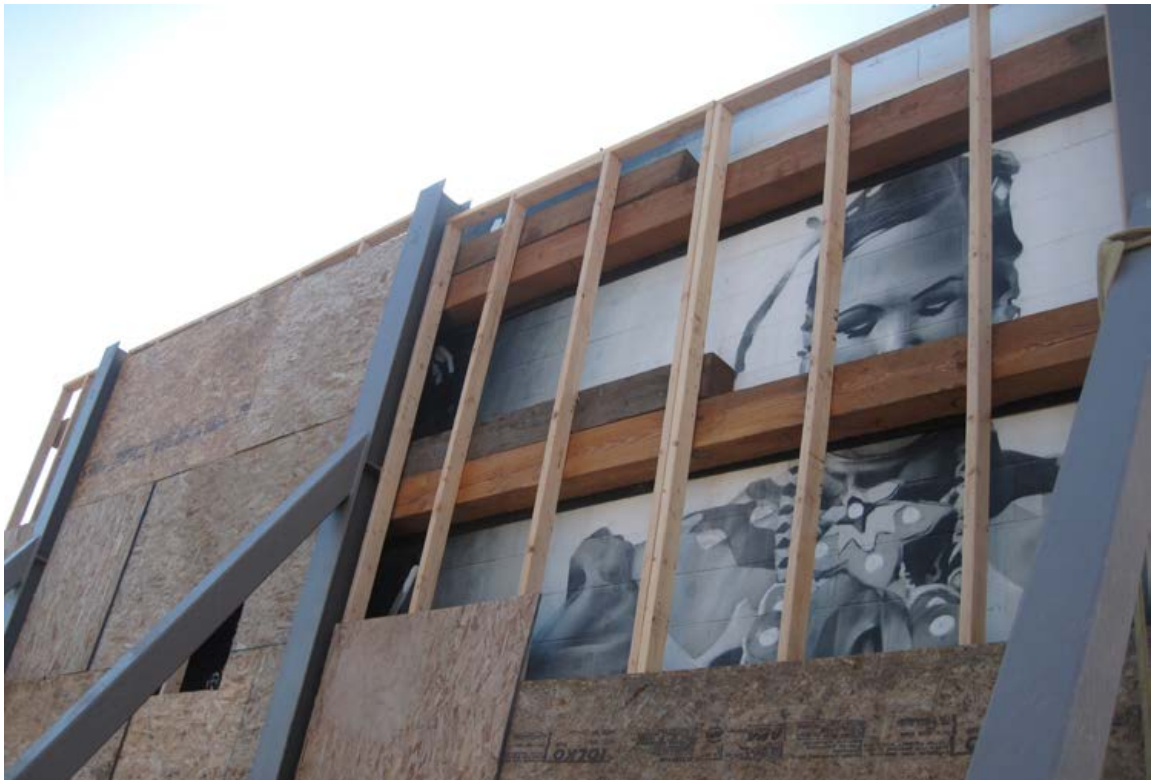
Plywood wall beign constructed on the face of the mural for added protection
