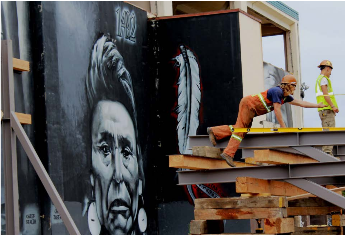
Assembly of the steel A-frames before they are put into place
