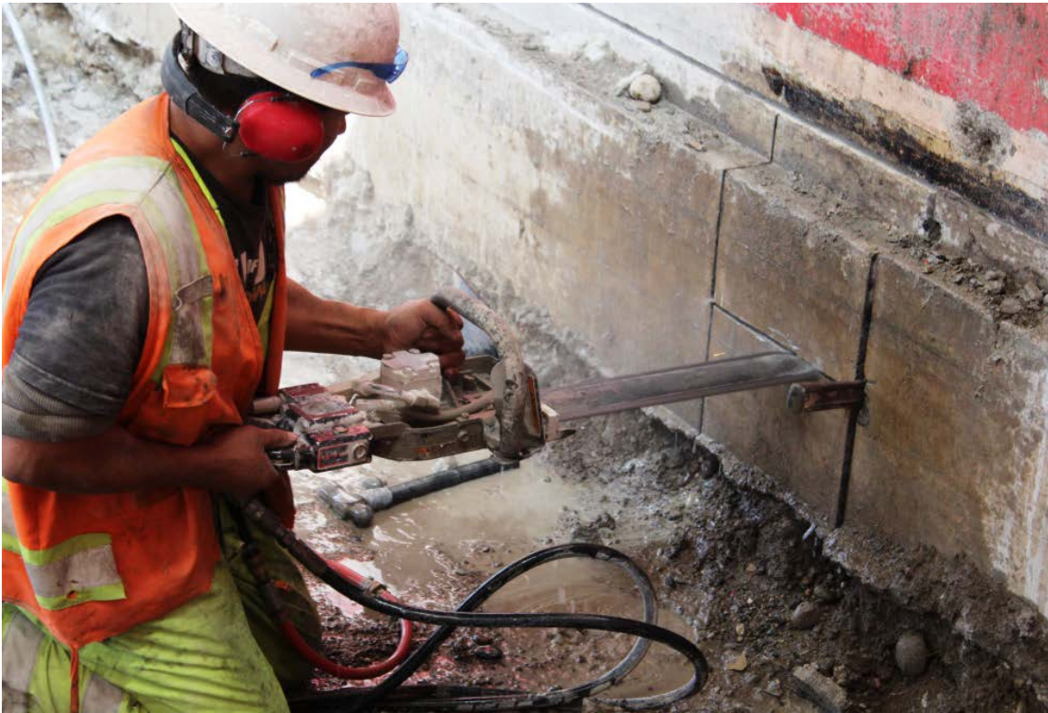
Evergreen Concrete Cutting, Inc. cutting through the wall
