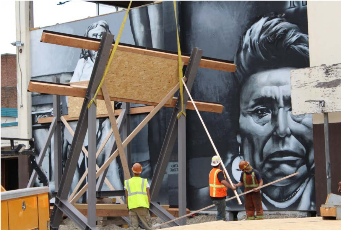
installation of the A-frames were lifted into place by a crane
