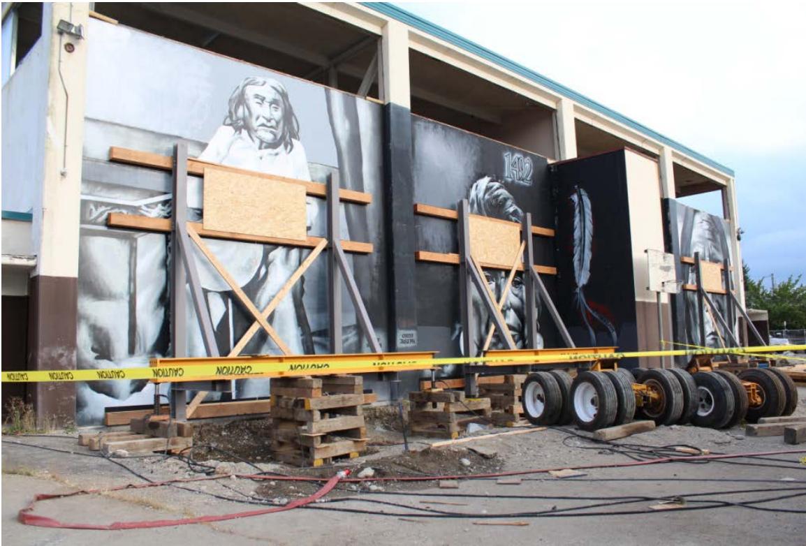
Hydraulic dollies ready to be attached to the A-frames for the removal of the murals
